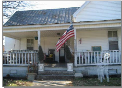
Historic homes shape the character in the Town Neighborhood character area of Varnell.
